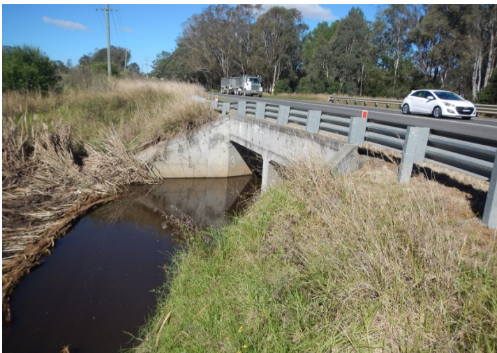
Badgerys Creek crossing at the Northern Road
