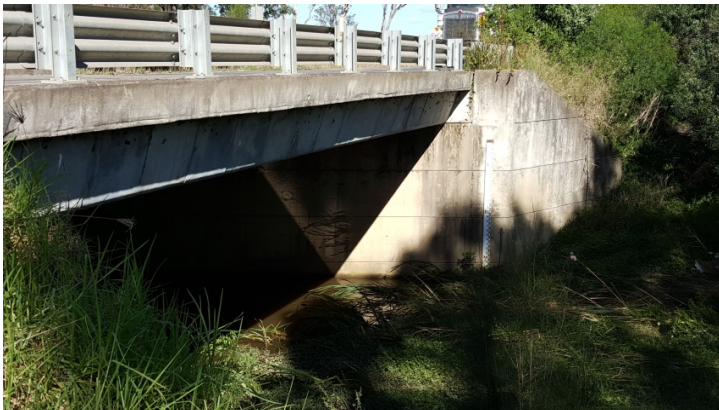
Badgerys Creek crossing at Badgerys Creek Road
