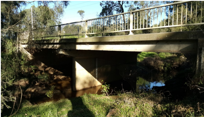
Badgerys Creek crossing at Elizabeth Drive
