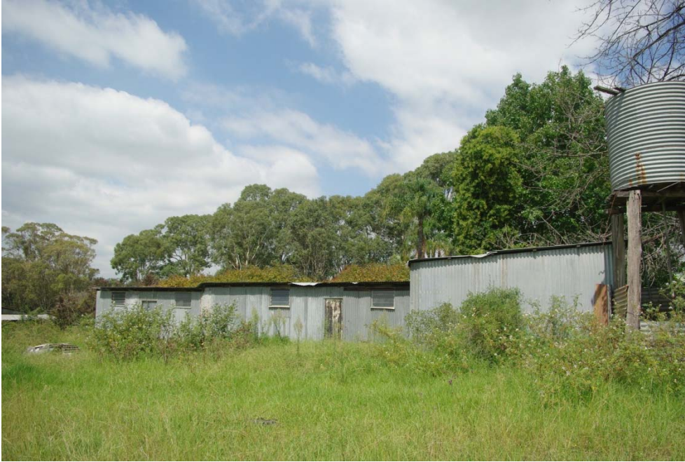
Plate A15 View south toward outbuildings. (Source: RPS 2015)
