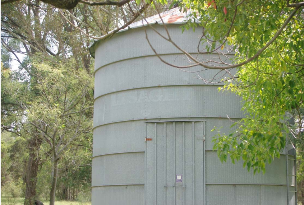
Plate A11 Lysaght silo. (Source: RPS 2015)
