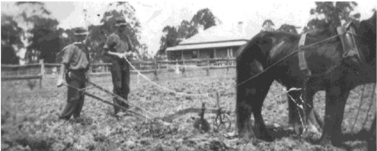
Plate 6 Ploughing on Nobbs' farm at Badgerys Creek in the 1940s. Note the hipped roof, bullnose veranda homestead, Exeter House, in the background. (Source: Liston 2009:46).
