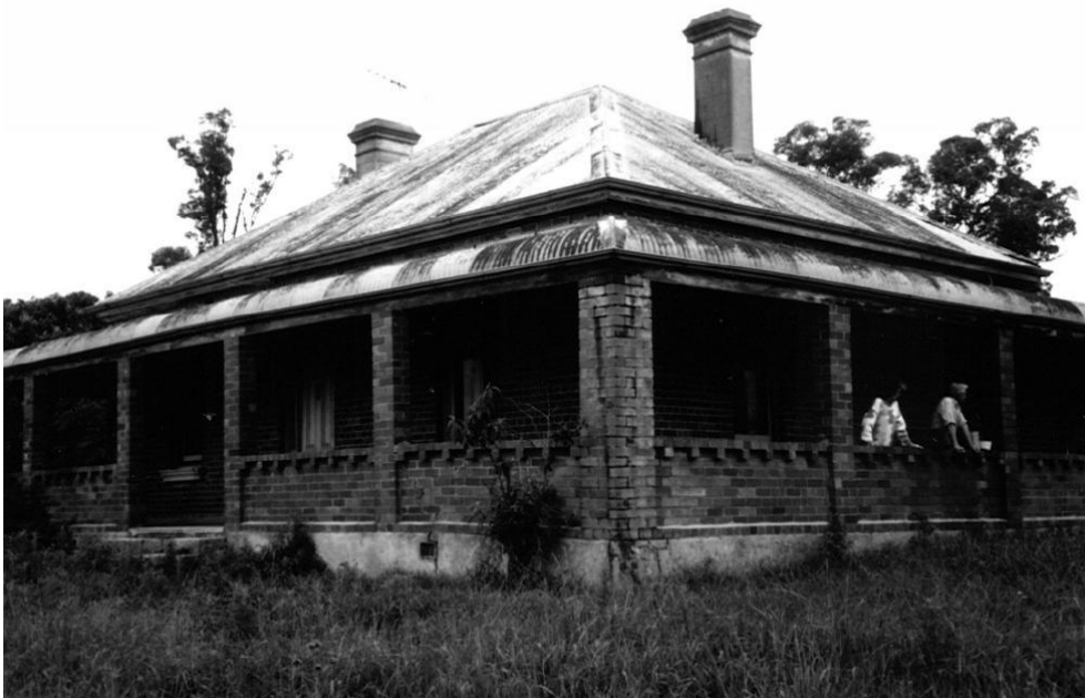
Plate 2 Photo of the substantial brick Exeter Farm house, originally constructed by James Badgery. Photography was taken in 1995 before the house was demolished. (Source: Liverpool City Library, Heritage Library Collection, 1776-12).
