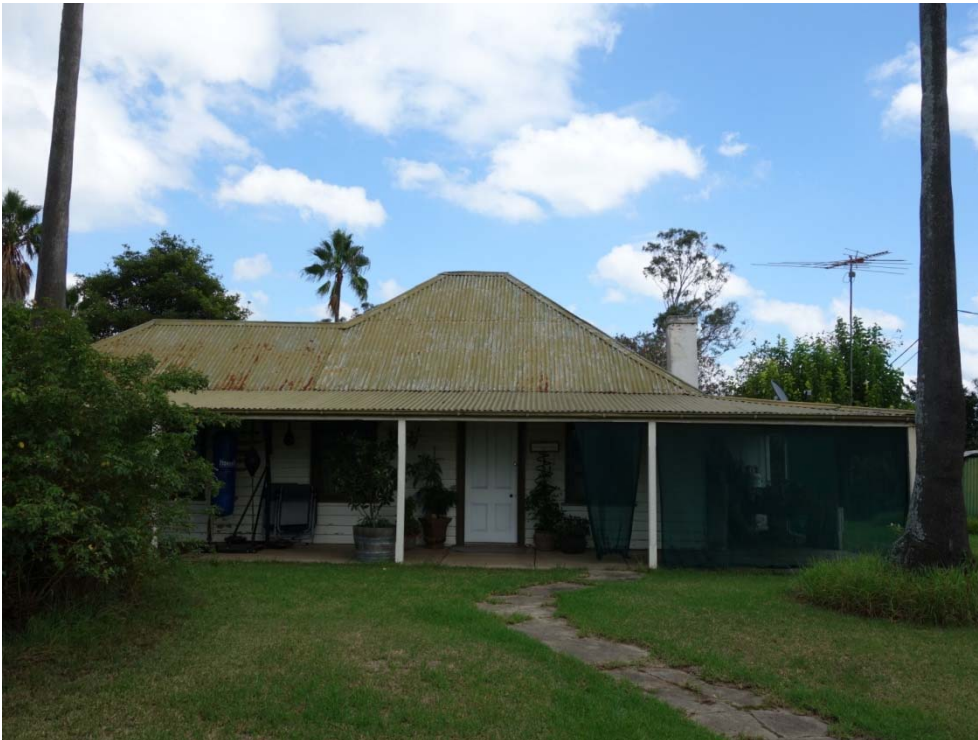
Plate A47 Vicary's Winery front of c.1860 slab homestead. (Source: RPS 2015)
