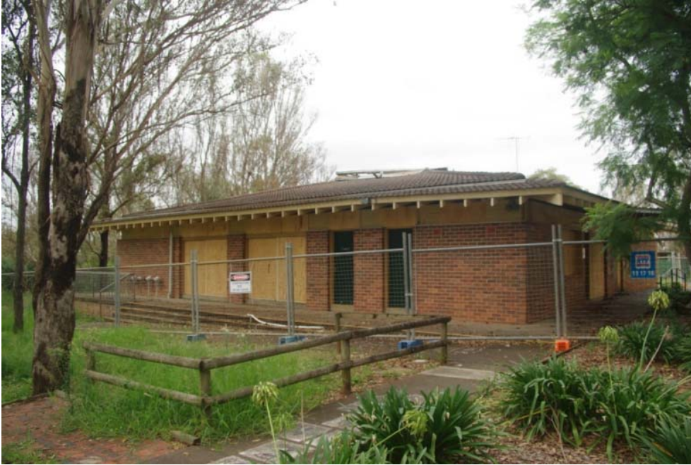
Plate A18 View south east toward classroom block. (Source: RPS 2015)
