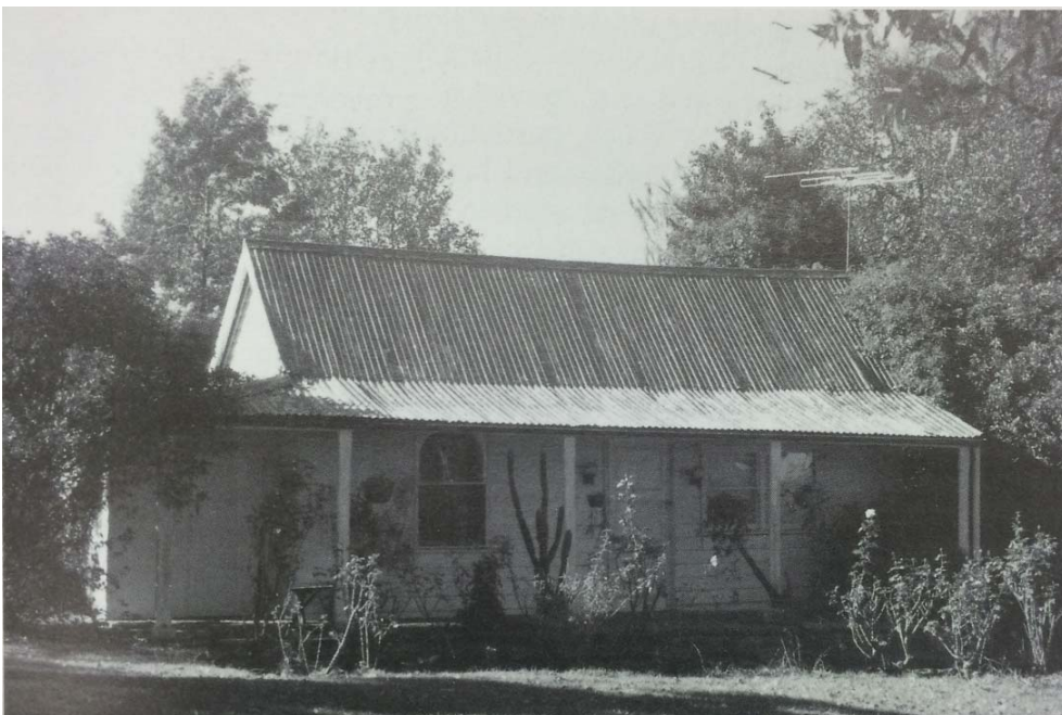
Plate A6 Ralph Wiener's residence. (Source: Donald and Gulson 1996:31)
