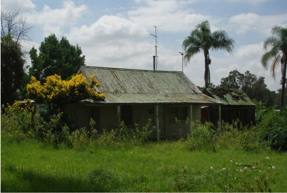
Plate A7 View north toward the cottage. (Source: RPS 2015)
