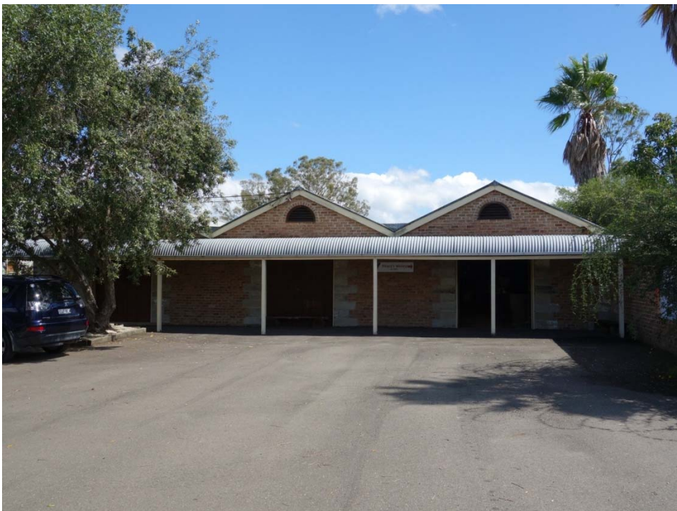
Plate A42 Vicary's Winery cellar door building. (Source: RPS 2015)
