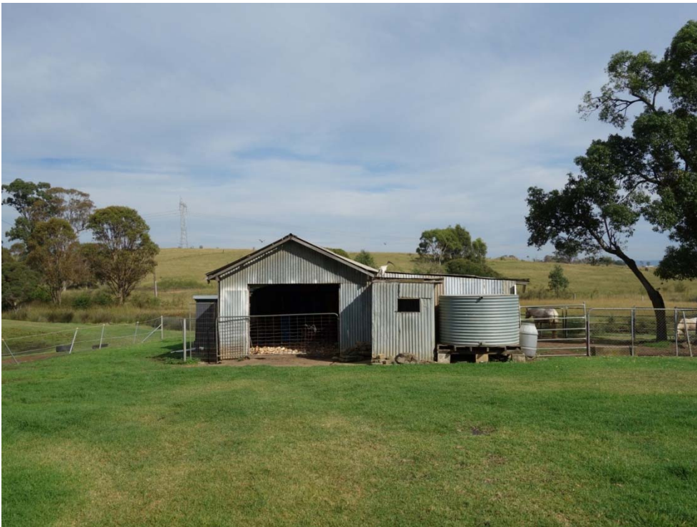
Plate A63 Lot 2 Jackson Road farm shed with accretions. (Source: RPS 2015)
