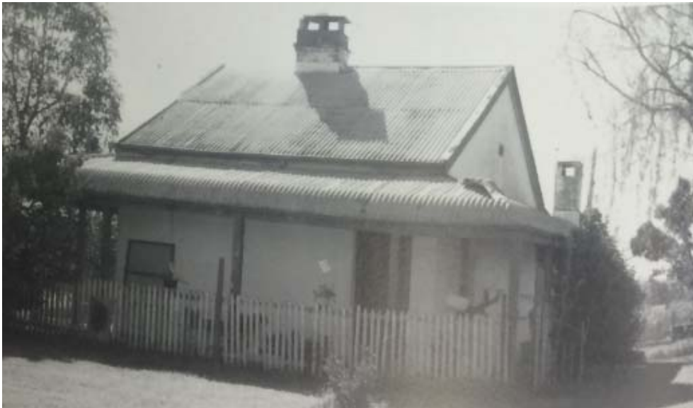
Plate A61 Undated photograph of house at Lot 2 Jackson Road. (Source: Donald and Gulson 1996)
