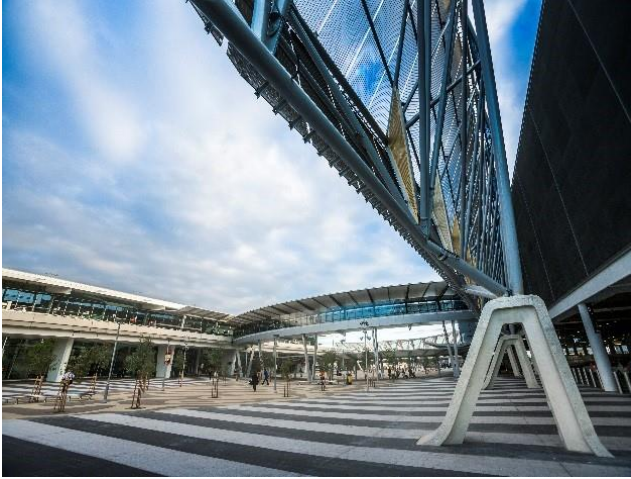
Figure 12. A high-quality, landscaped airport entrance and terminal precinct — Adelaide Airport.
