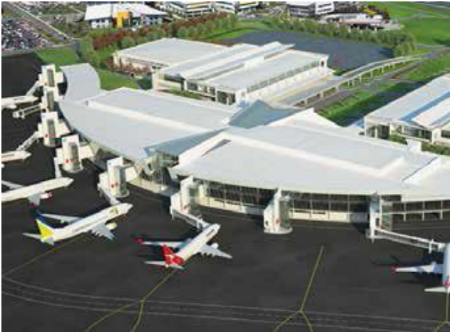
Figure 53. Aerobridges as an extension of the overall design — Canberra Airport.
